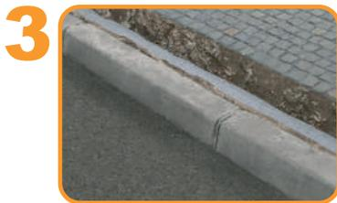
Proceed with the concrete cast for creating the laying bed and wait that the concrete has reached the right consistency (one hour at least).
