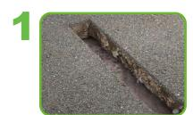
Realize the excavation according to the dimensions required in the project. The dimension will be on the diameter of the required pipe.
