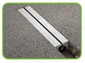
Cover the cones and the pipe with concrete with resistance class according to the class of load requested.
